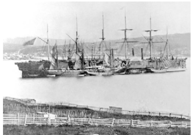
The new transatlantic cable was laid by the ship Great Eastern captained by Sir James Anderson. Her immense hull was fitted with three iron tanks for the reception of 2,300 nautical miles of cable (PD).
