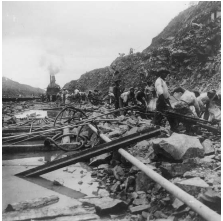
Construction of the Canal, 1909
