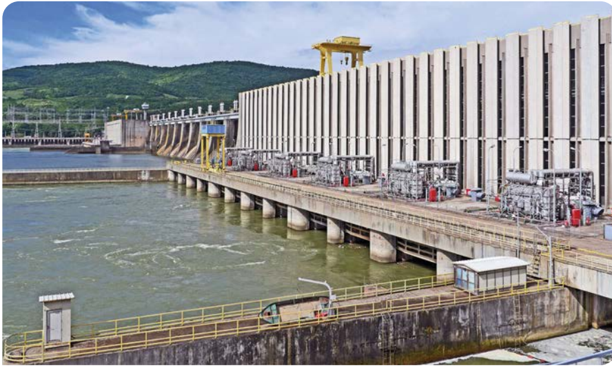
Iron Gate I Hydroelectric Power Station, the largest dam on the Danube river and one of the largest hydro power stations in Europe
