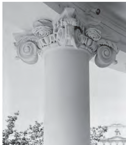
Capital of a Column on the Truman Balcony
