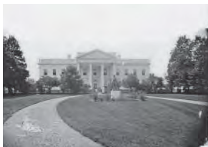
Historic Photo Showing North Portico
