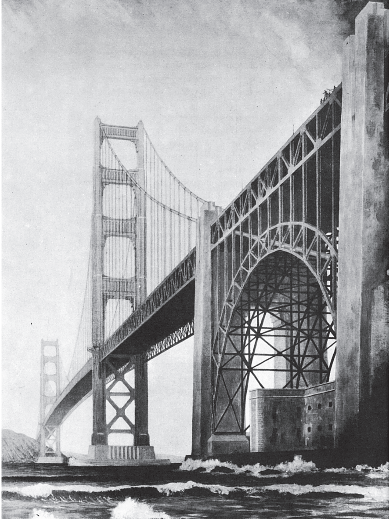
One of the steel spans of the Golden Gate Bridge arches protectingly over old Fort Winfield Scott. This fort was built in 1854 at a point where the Golden Gate is narrowest. It was in this fort that the commander's ten-year-old son, Sydney Taylor, Jr., in 1879, stuffed the biggest cannon so full of charcoal dust that it was unable to fire a salute when General U. S. Grant passed by.
